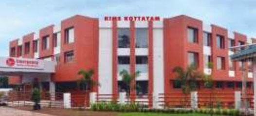
KIMS Health Hospital, Kottayam, India
